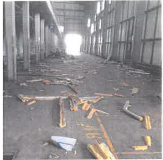
Photo 6 Metals stripped from building
