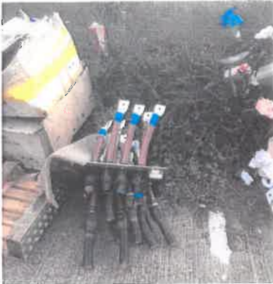
Photo 5 Metals stripped from building
