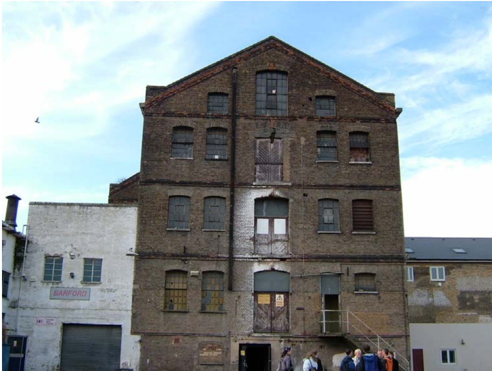
Figure 23 the Granary in 2008. It is five storeys high and quite dominant on Abbey Road. The architecture is similar to that of the Malthouse (source: the writer)
