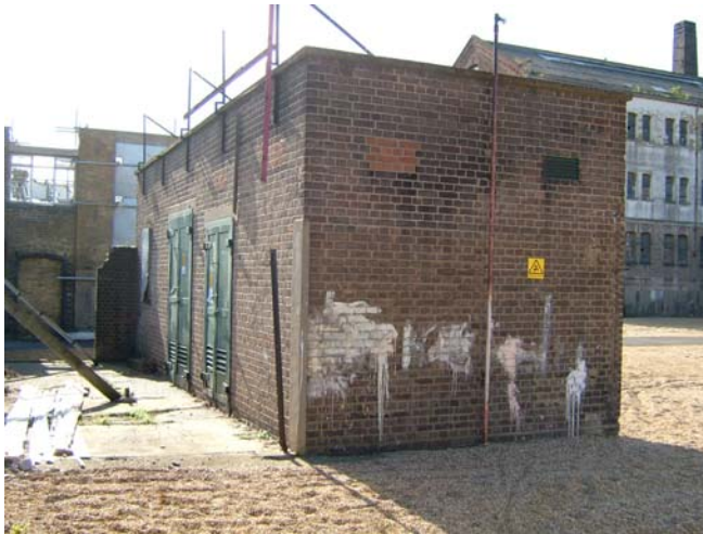
Figure 34 sub-station near the Abbey Road frontage (source: the writer)
