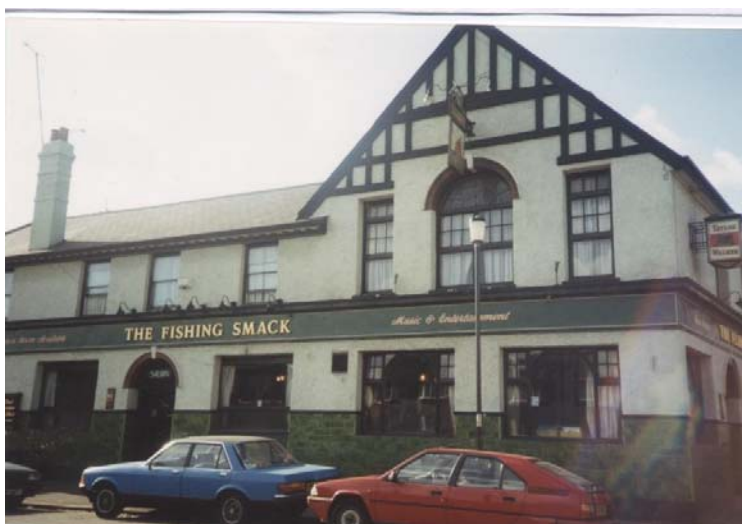
Figure 33 the Fishing Smack showing the rebuilt façade and extension (source: the writer)
