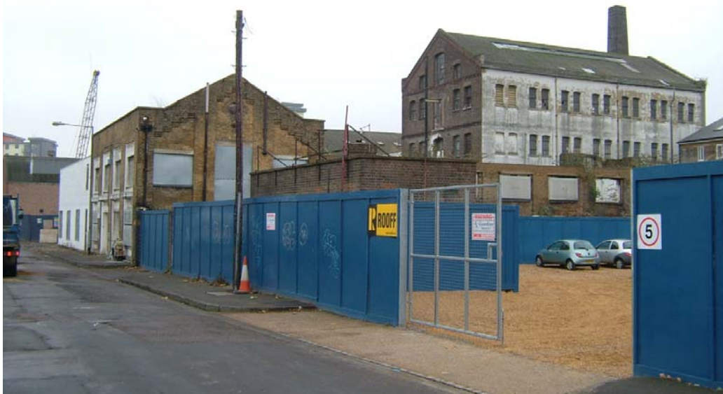
Figure 28 the two storey Malthouse Extension before it was demolished (Granary the taller building behind) (source: the writer)
