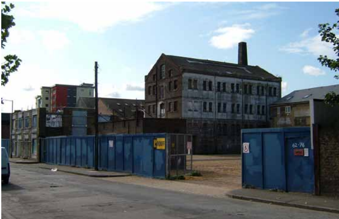
Figure 17 view of the conservation area today from Abbey Road showing the Malthouse and Granary building as the main remaining features (source: the writer)
