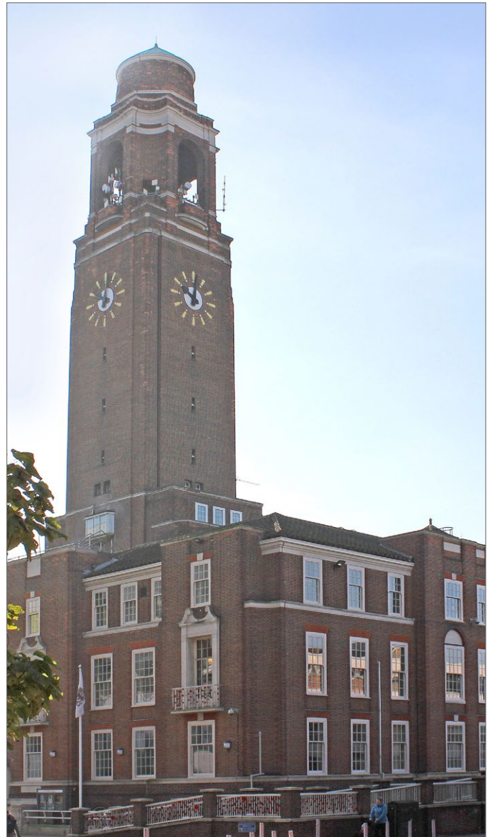
Barking Town Hall, a locally listed building and the civic heart of the town
