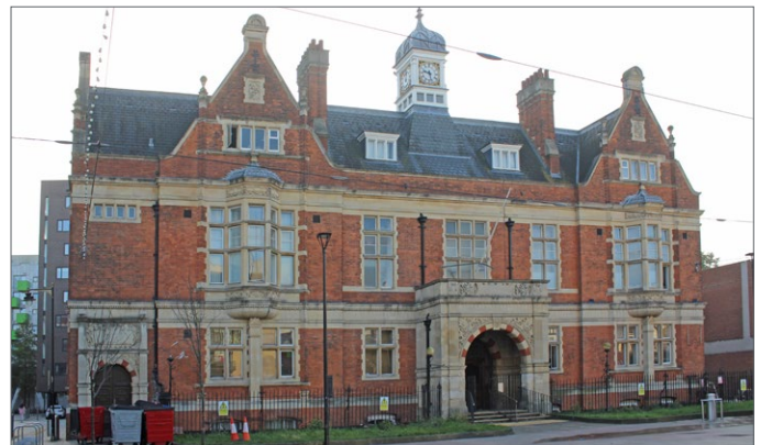
The former Magistrates Court has lots of decoration and is one of the grandest buildings in the conservation area
