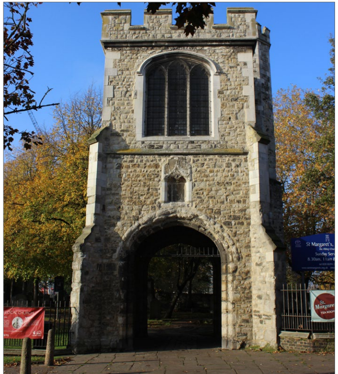
The medieval Curfew Tower is one of the few buildings in the conservation area to be constructed in stone
