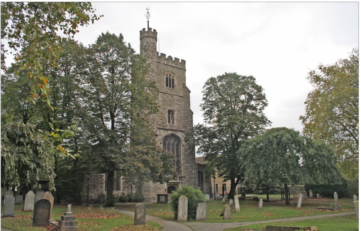
All older buildings in the conservation area require regular maintenance including the medieval St Margaret's Church
