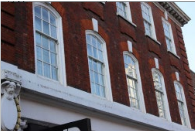
White painted timber-framed sash windows in the conservation area
