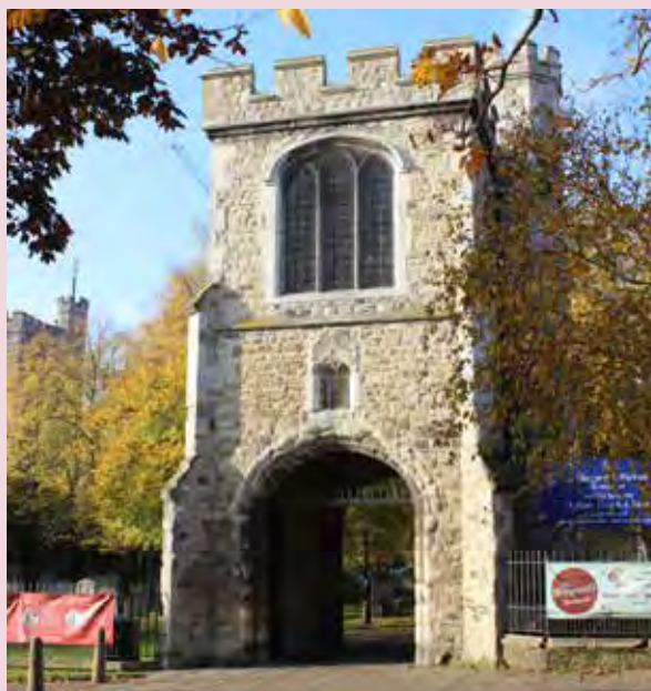
The Curfew Tower is the only surviving building of Barking Abbey.
