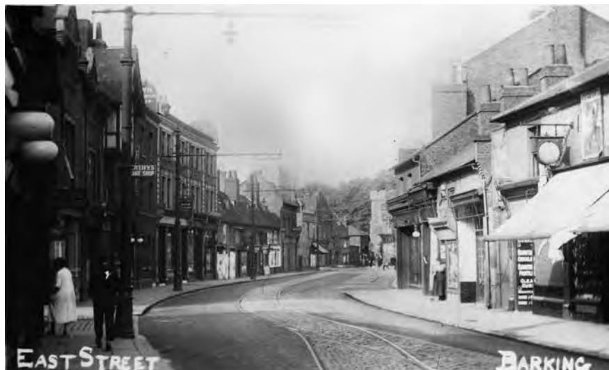
This shows East Street looking south-west. The south side of East Street is completely unrecognisable owing to the negatively-contributing modern shops, which replaced the former, more diverse mix of buildings. The Locally Listed 2a-4a East Street (former Burtons) had not yet been built. The Curfew Tower and the church tower are visible in the background. (Barking & Dagenham Archives and Local Studies, Valence House: DS385b)
