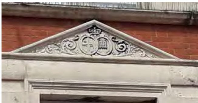
The crest of the United Westminster Charities Schools remains today in the pediment above each first-floor window.
