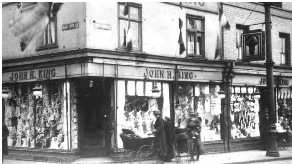
This Victorian shopfront (John H. King) on the corner between East Street and the Broadway shows the building in place before the 1930s 2a-4a East Street (former Burtons). (Barking & Dagenham Archives and Local Studies, Valence House: HHL2621)
