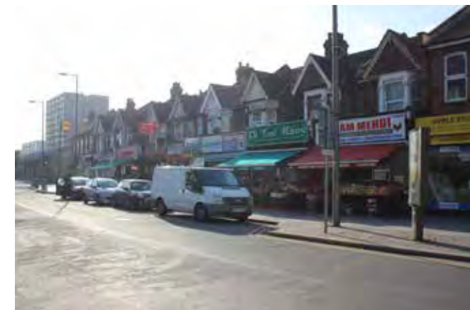
Two storey terraced buildings in Ripple Road.
