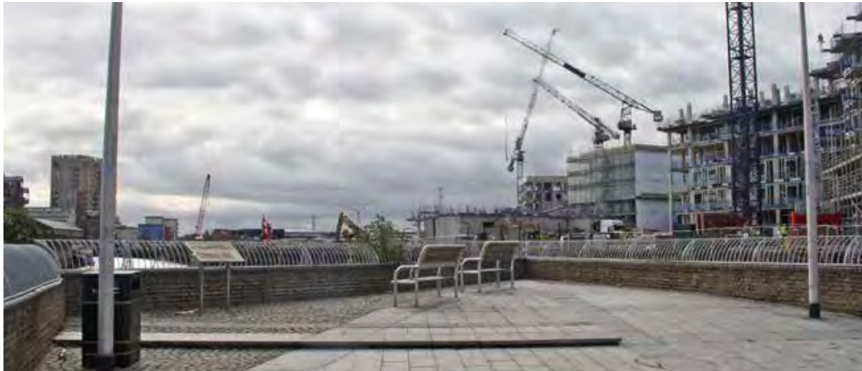
Public realm around the Town Quay
