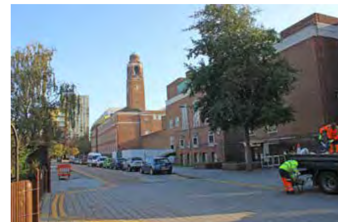
The clocktower of the three storey Town Hall is visible from across the conservation area.
