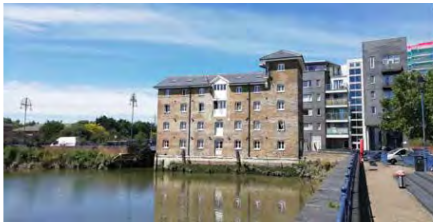
The Old Granary, the only building within this sub-character area and reminiscent of the warehouses which would once been prevalent in this part of the town'
