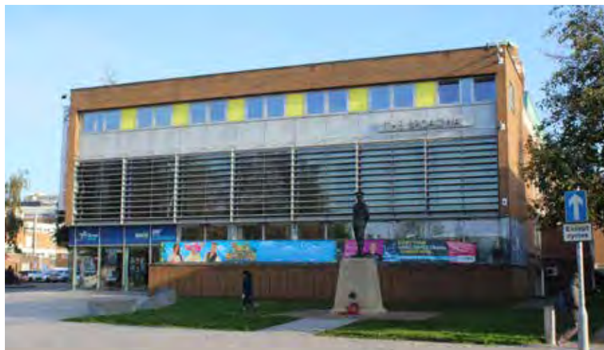
More recent buildings of larger massing and grander proportion; shown here are the Town Hall and Broadway Theatre.
