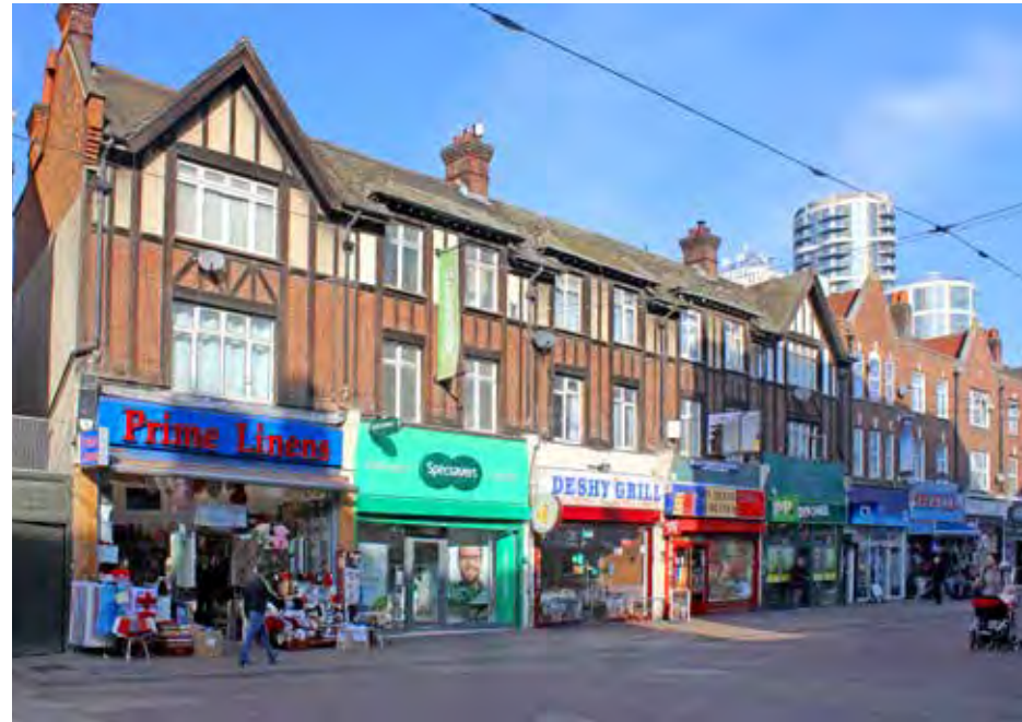
Typical three-storey terraced buildings along East Street.
