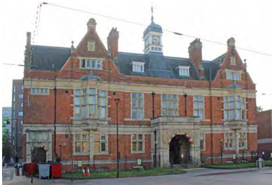
Barking Magistrates' Court is a landmark building for its highly decorative appearance and position at the heart of East Street.
