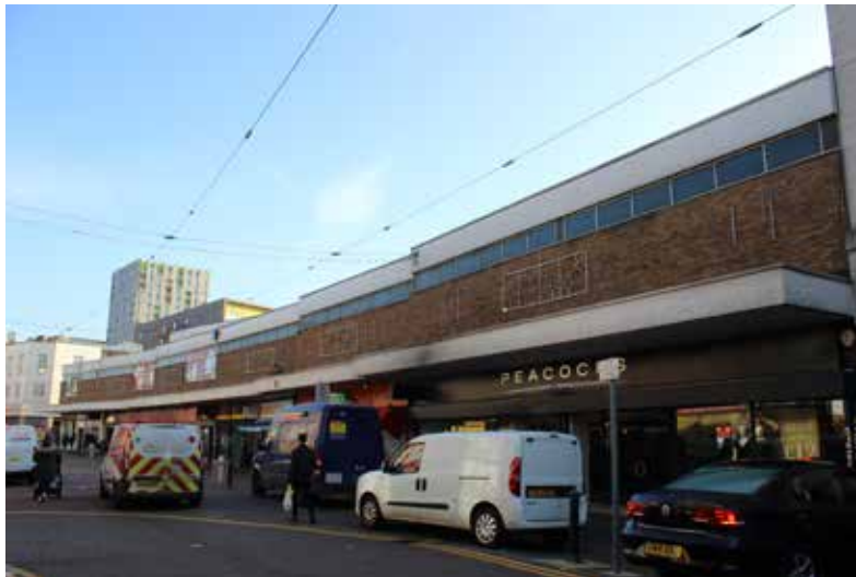
10-30 East Street is a detracting building.
