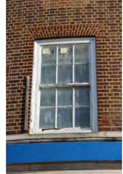
Many of the surviving timber windows are in a poor condition from neglect and lack of maintenance
