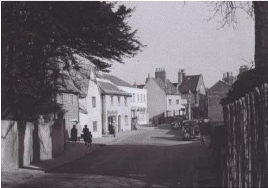
Figure 2 looking east along Crown Street in 1952 from the location of the vicarage (source: Curtis, S. Gillespie, G. Clifford, T. You've Never had it so Good A photographic record of Dagenham in the 1950's London: Borough of Barking and Dagenham page 9)
