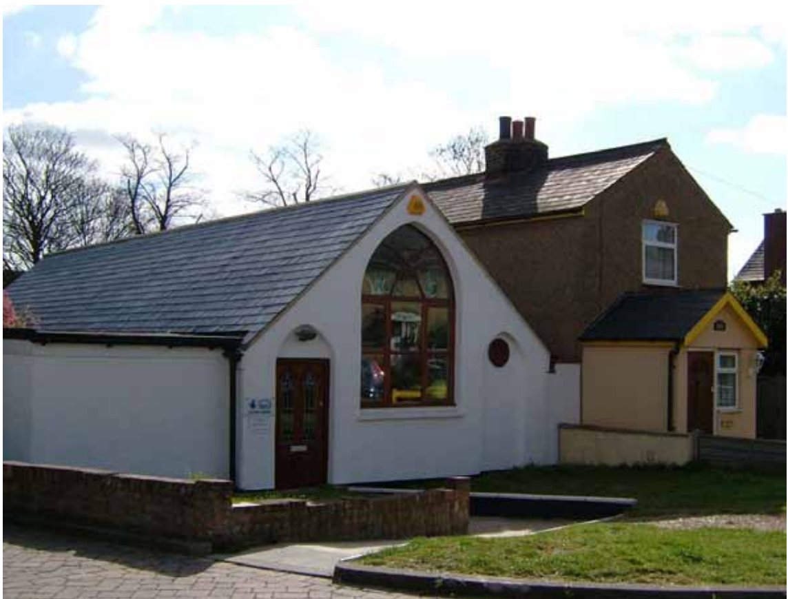
Figure 17 the Dagenham Old National School has been restored
