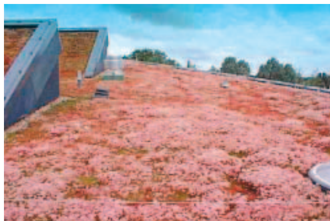
Extensive Green Roof with sedum, Great Notley Primary School (Photo: Bauder Ltd)
