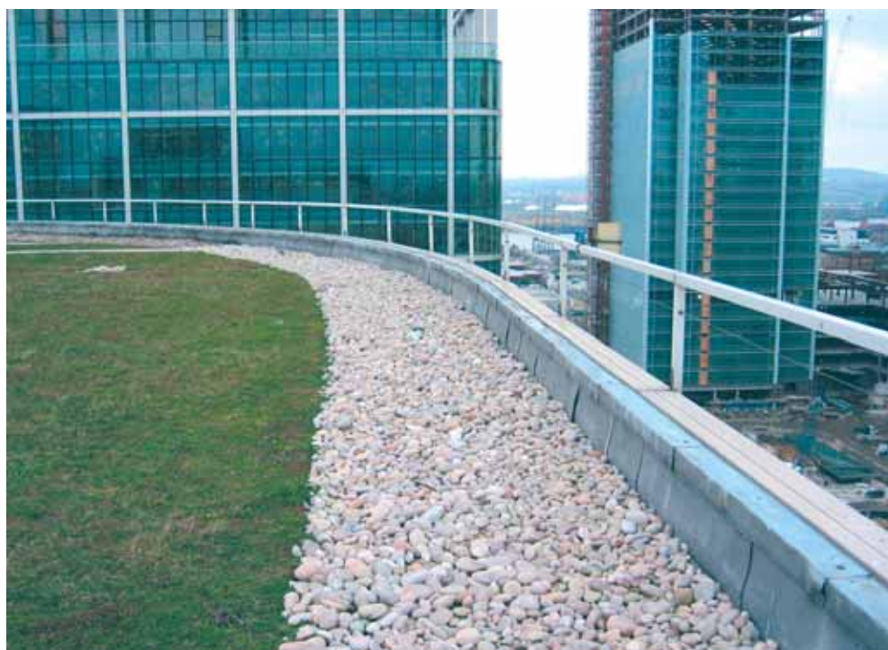
Extensive Green Roof at Canary Wharf (Photo: Dusty Gedge)
