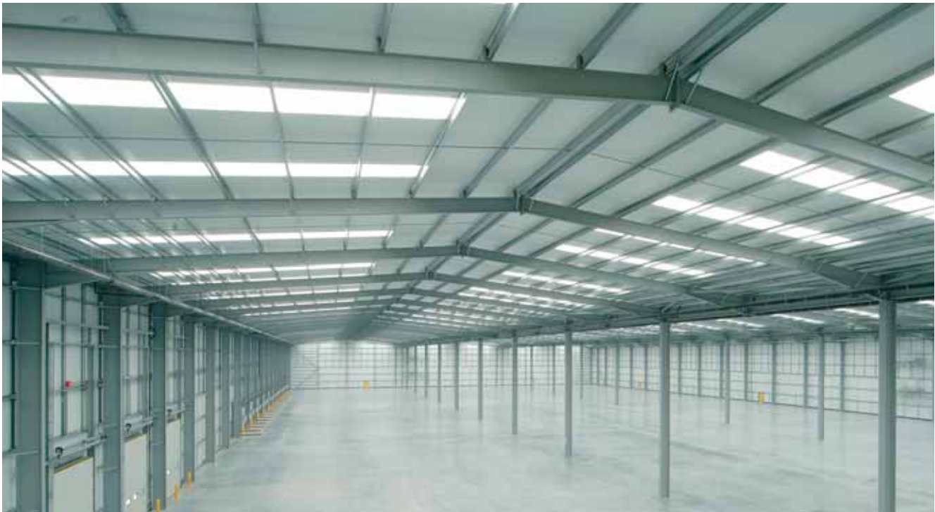
The Voltaics warehouse in Dagenham Dock makes the most of natural light through roof design.
