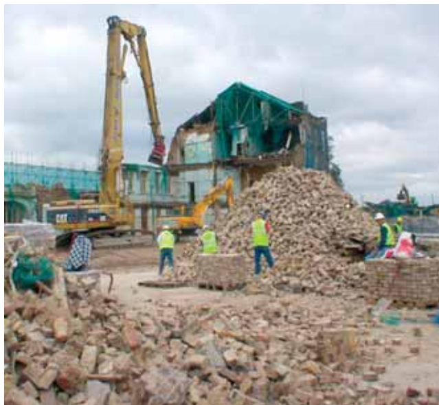
Bricks being segregated on a demolition site so they can be reused. (Photo: EnviroCentre)
