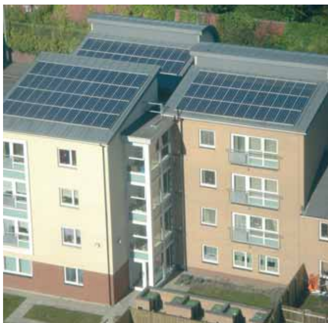
Queens Cross Phase 2 in Glasgow integrates photovoltaics on the roof. (Photo: solarcentury.com)
