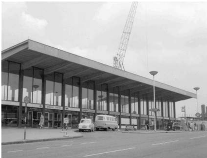
Figure 8: Barking Station shortly after completion in 1961
