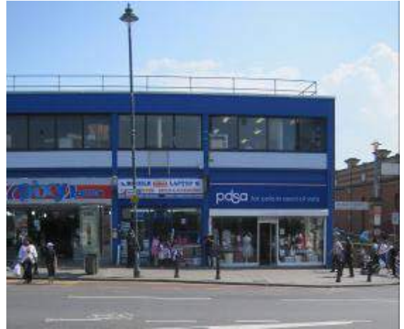
Poor quality building stock does not have a positive impact on the character of Station Parade.
