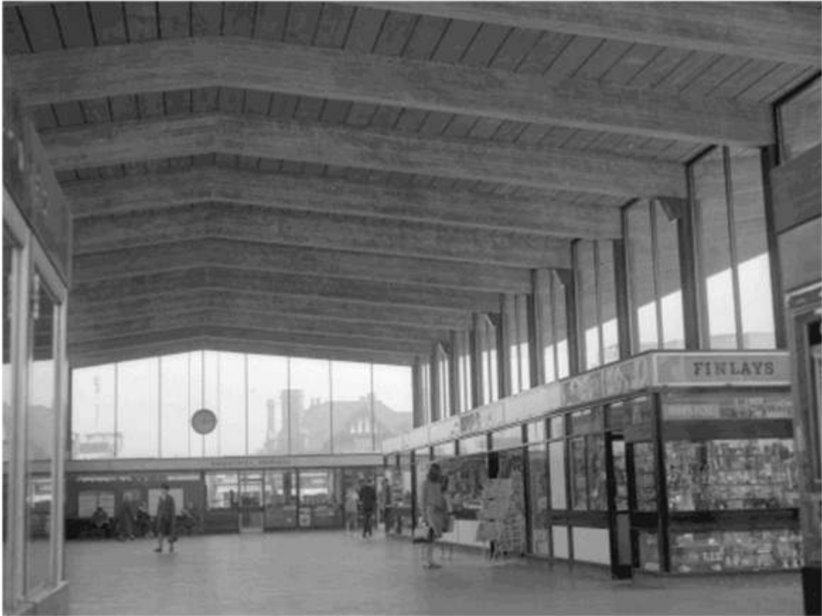
Figure 9: An internal view of Barking Station, around 1961
