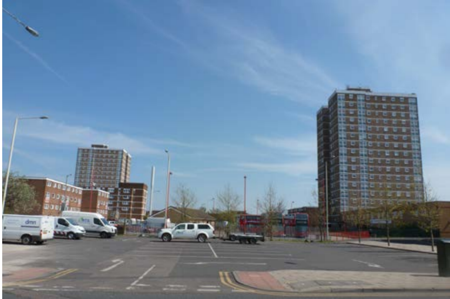
Site 4: view east towards the Civic Centre
