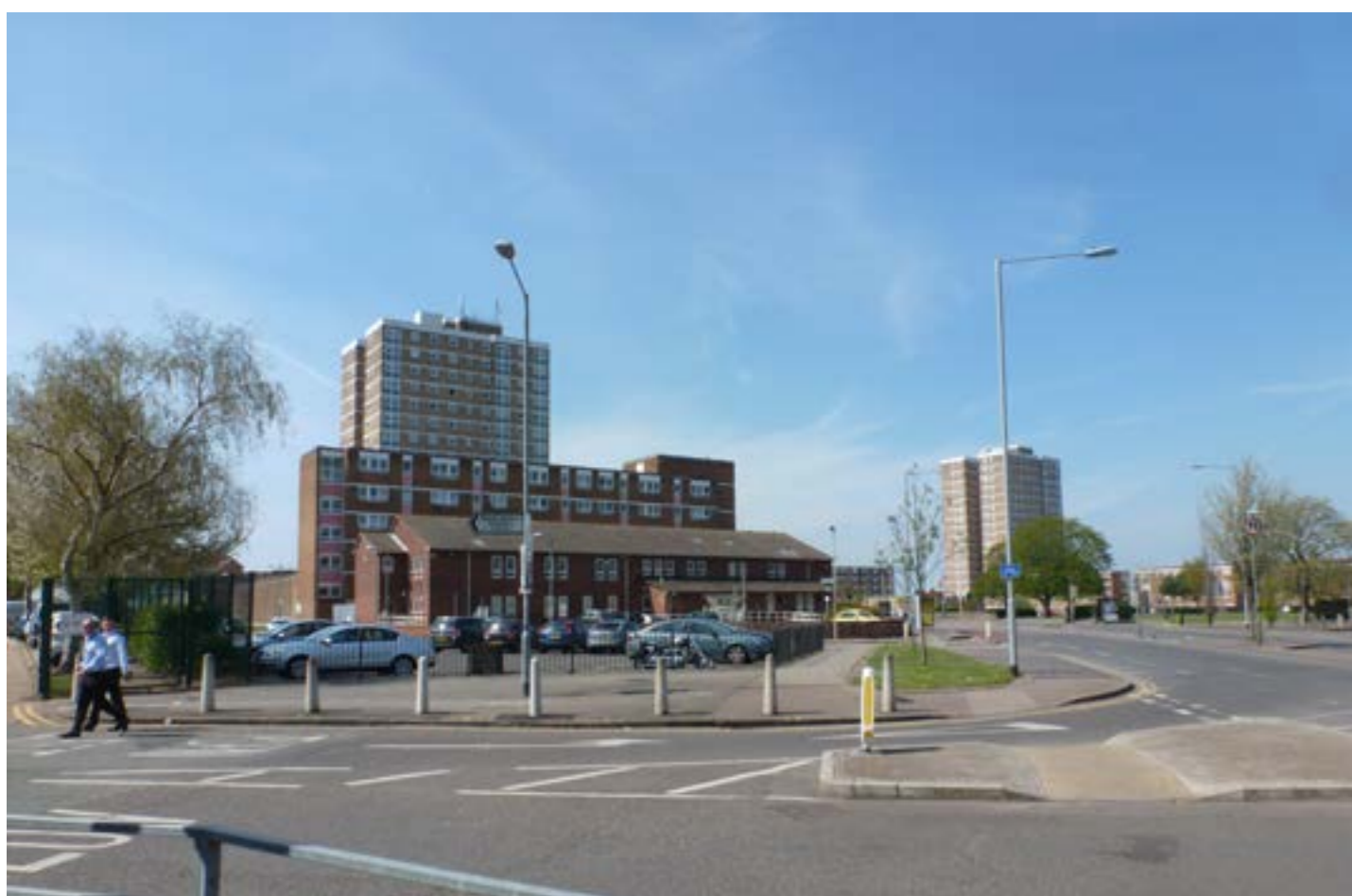
Site 9E: view towards the site from Rainham Road
