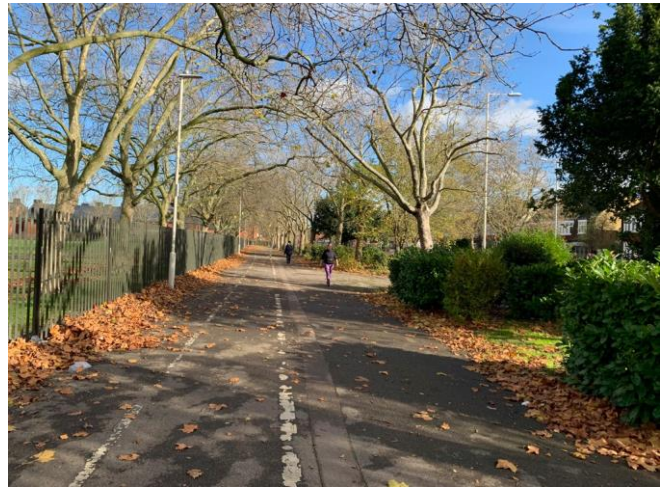
This shared use path, by Barking Park, doesn't comply with the latest national cycling design guidance.
