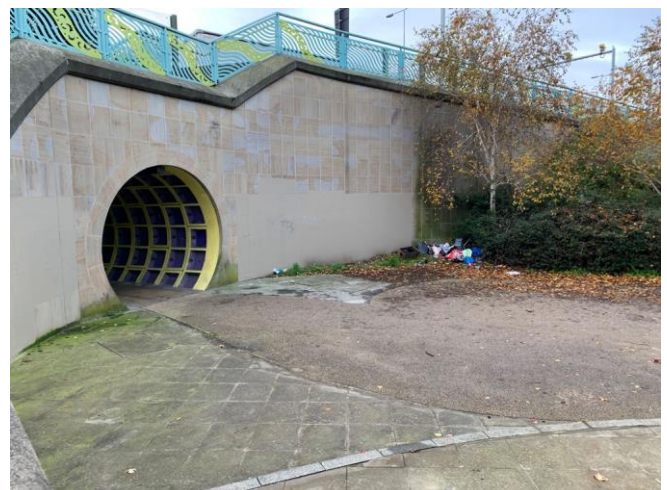
This subway and approaches, under the A13 at Alfred's Gardens, are unwelcoming, especially after dark.
