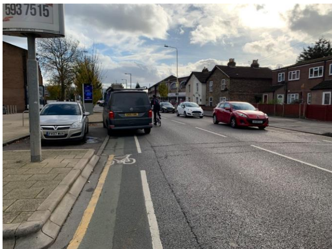
Advisory cycle lanes are often parked in, and this one also needs to be crossed to access the parking bay.
