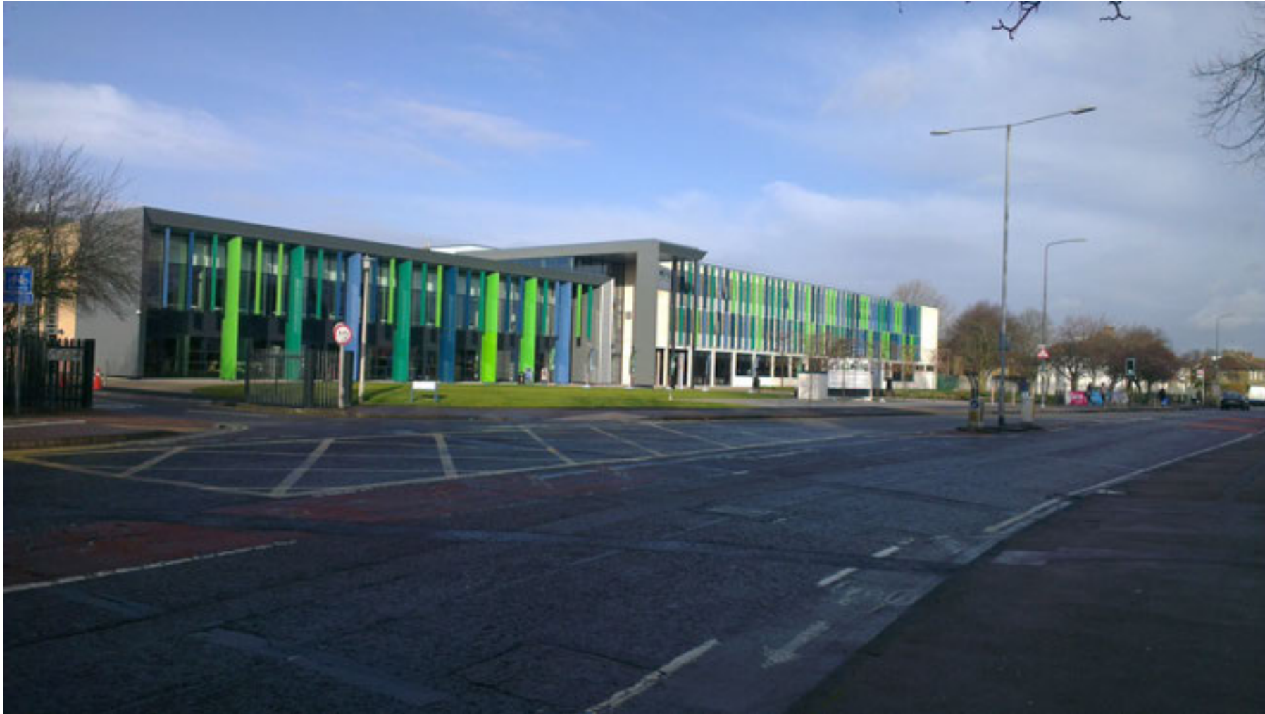
Figure 1: TEG Organic Waste Treatment Centre, Choats Road, Dagenham.
