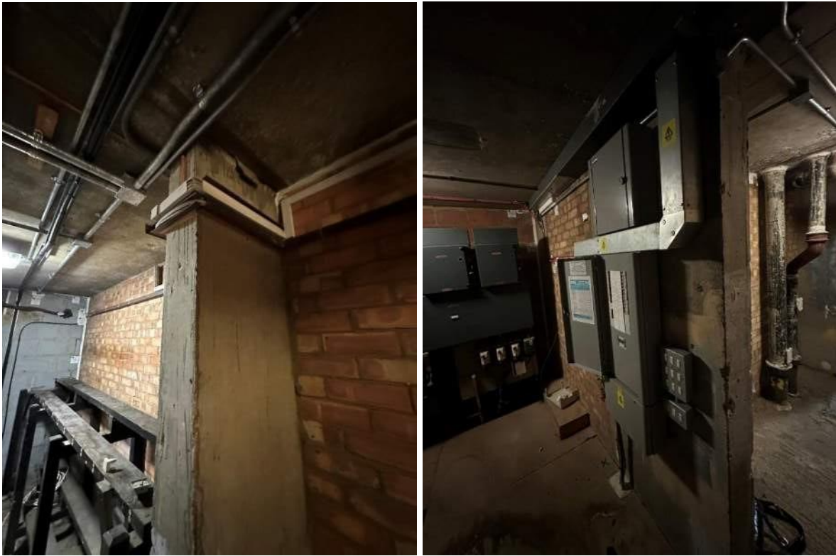
Figure 16 and 17: Vertical RC Structure Visible with RC soffit
